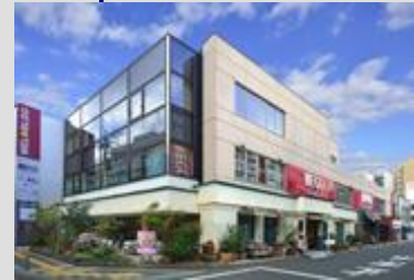
MEL Building (Sendai-shi, Miyagi Pref.)
