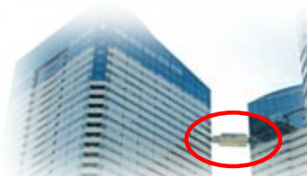
Connecting vibration control bridge
