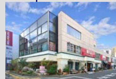
MEL Building (Sendai-shi, Miyagi Pref.)
