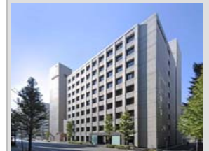
Kanda Nishiki-cho 3-chome Building (formerly called Sumitomo Corporation Nishiki-cho Building)
