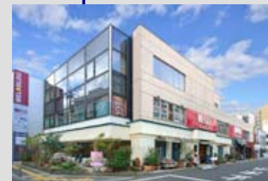
MEL Building (Sendai City, Miyagi Pref.)
