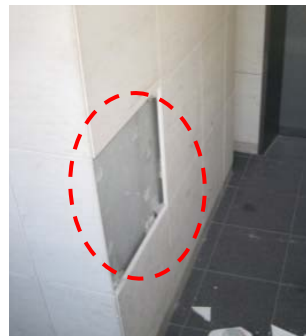
PRIME URBAN Nagamachi Icchome (chipped wall in common area)
