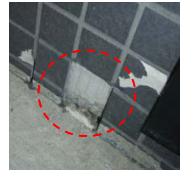
PROUD FLAT Asakusa Komagata (exterior tile detachment)
