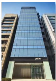
PMO Nihonbashi Odenmachi (Chuo-ku Tokyo)
