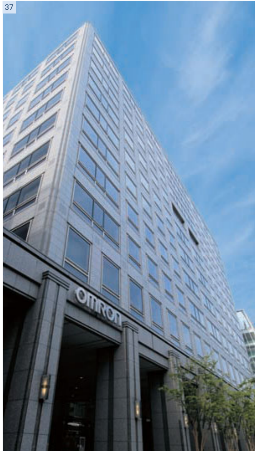
37 | Omron Kyoto Center Building
