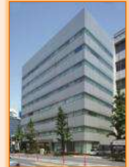
NF Hongo Building
