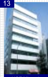
NOF Minami- Shinjuku Bldg
