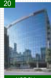
NOF Shin- Yokohama Bldg
