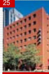
NOF Midosuji Bldg
