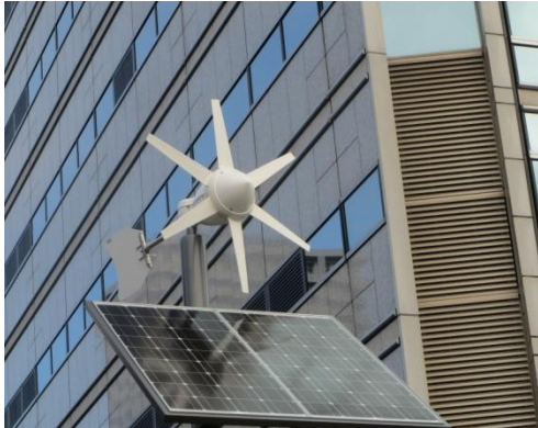
Installation of wind power generator and solar power generator
