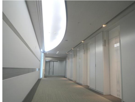
Installation of LED light bulbs
