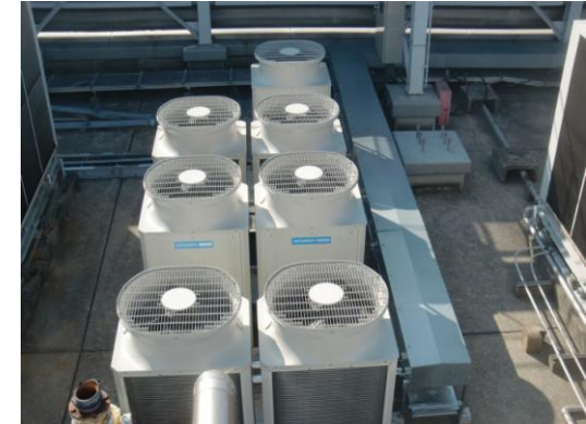
Renewal work of air-conditioning system
