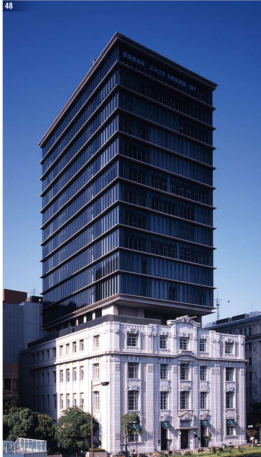
48 | NOF Kobe Kaigan Building
