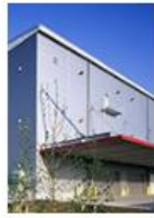
Atsugi Minami Logistics Center B Tower
