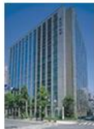
NRE Osaka Building
