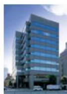
NMF Aoyama 1-chome Building
