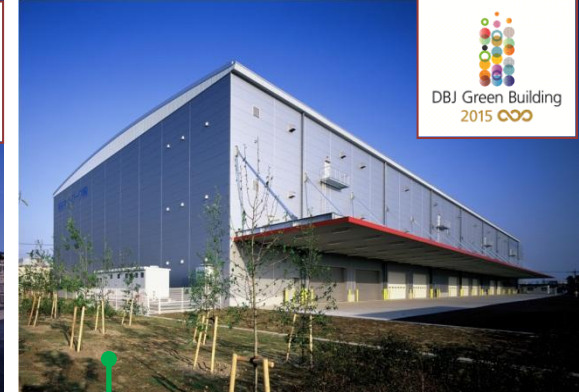
Atsugi Minami Logistics Center B Tower
