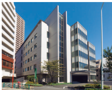
NMF Shinjuku EAST Building
