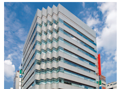
NRE Ueno Building
