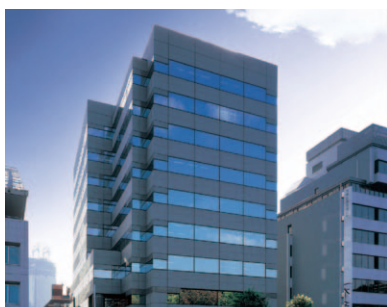
NMF Aoyama 1-chome Building
