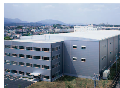
Atsugi Minami Logistics Center B Tower
