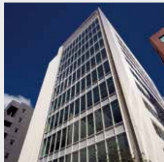
NRE Sapporo Building
