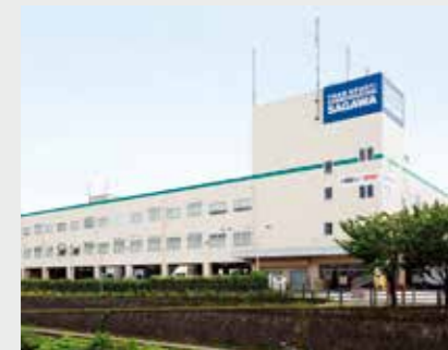
Kawaguchi Logistics Center A Tower
