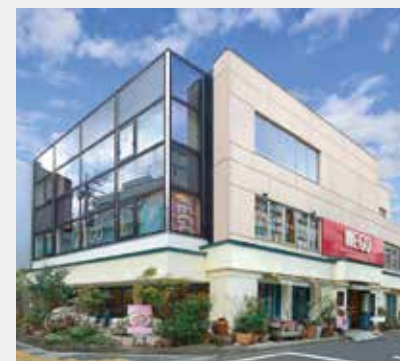
MEL Building Location: Sendai City, Miyagi Total floor area: 1,756.32 m 2
