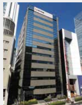
NRE Nishi-Umeda Building Location: Osaka City, Osaka Total floor area: 8,036.71 m 2
