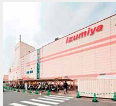
Izumiya Senrioka Location: Suita City, Osaka Total floor area: 24,399.12 m 2
