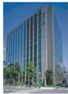
NRE Osaka Building
