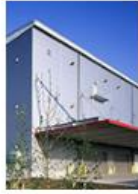
Atsugi Minami Logistics Center B Tower
