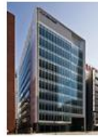
NRE Sapporo Building
