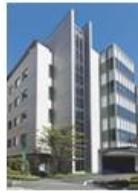
NMF Shinjuku EAST Building
