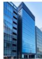
PMO Tamachi Higashi
