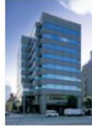
NMF Aoyama 1-chome Building
